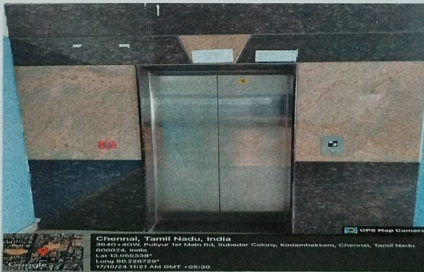
Figure 5. Lift facility in Mechanical Block
