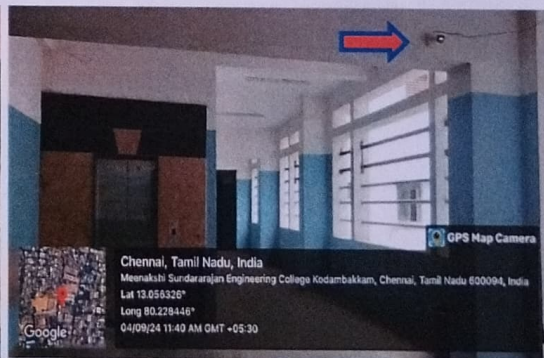
Fig. 7. : CCTV Camera at Mechanical Block First Floor
