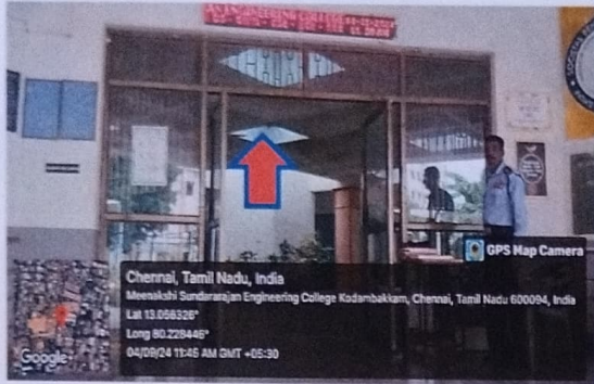
Fig. 2. : CCTV Camera at Main Block Entrance
