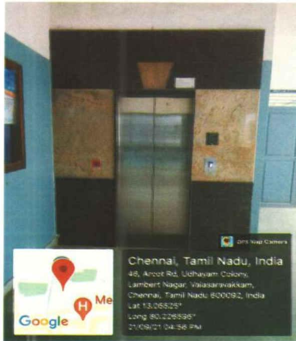
Figure 4. Lift facility in Sri Vidhushekhara Bharathi Block (civil block)
