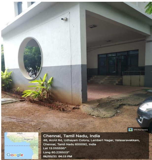
vii) CCTV Camera near parking zone
