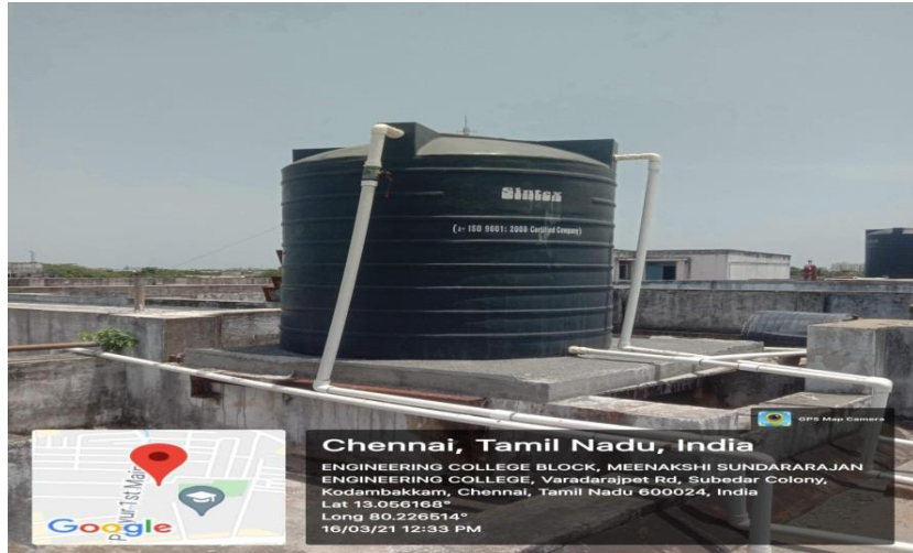
Fig. 5 : LOCATION: CIVIL BLOCK
