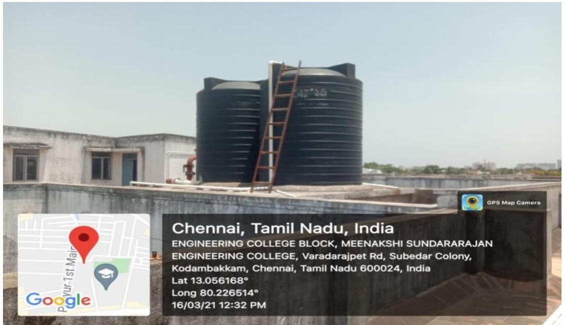
Fig. 7 : LOCATION: MECHANICAL BLOCK
