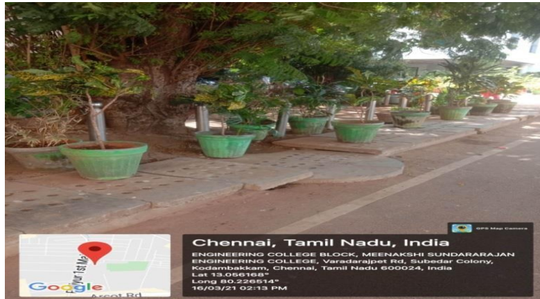
Fig. 2 : RAIN WATER HARVESTING
