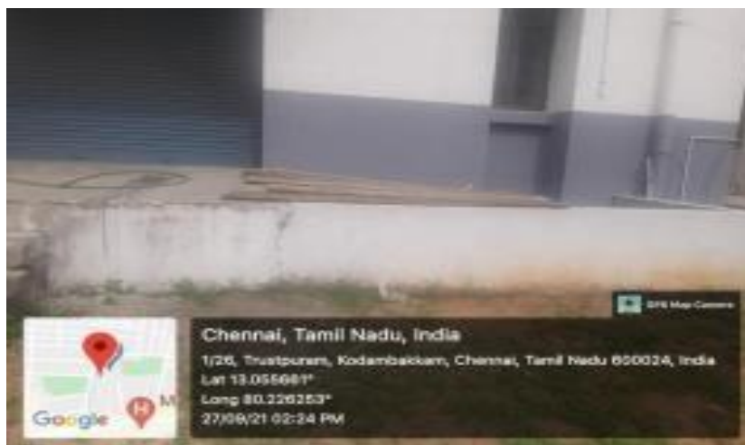
Fig. 2: Civil Block - Solid waste Management: Composting - Back side
