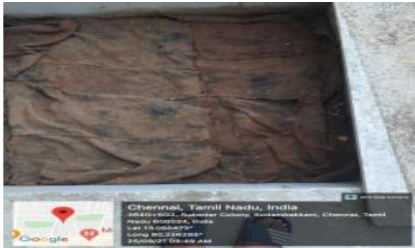
Fig. 3 : Civil Block - Solid waste Management: Composting - Back side
