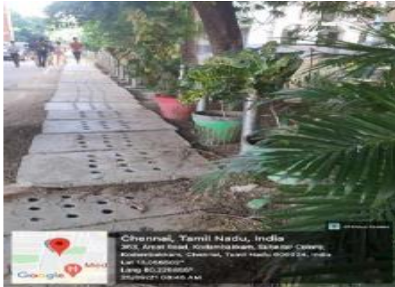
Fig. 6: Liquid waste Management: Effective rain harvesting system
