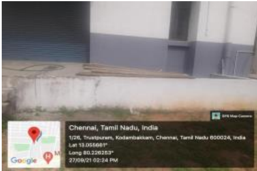
Fig. 2: Civil Block - Solid waste Management: Composting Back side
