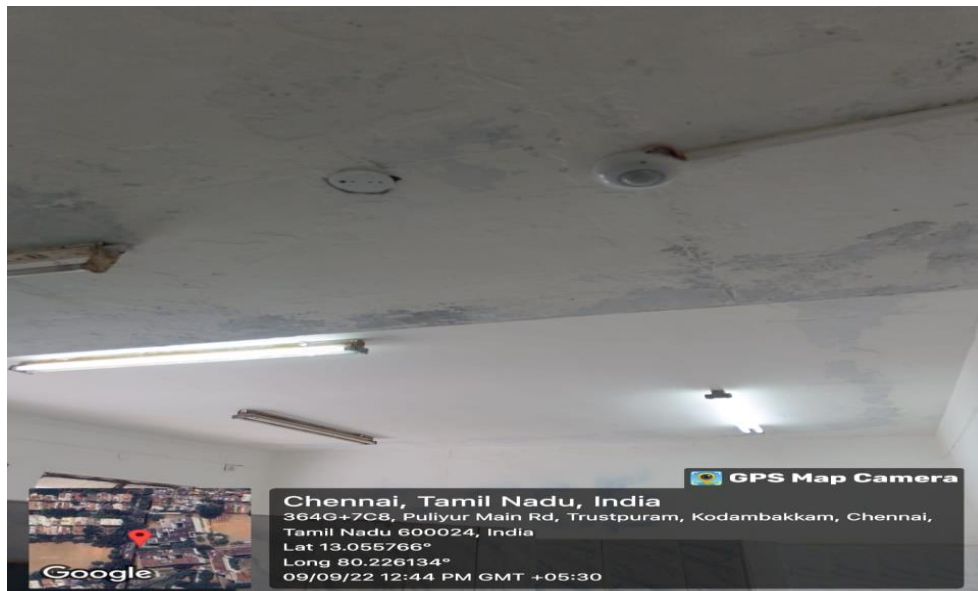
Figure5. Installed Sensor based Lights in Restrooms(Mech block)
