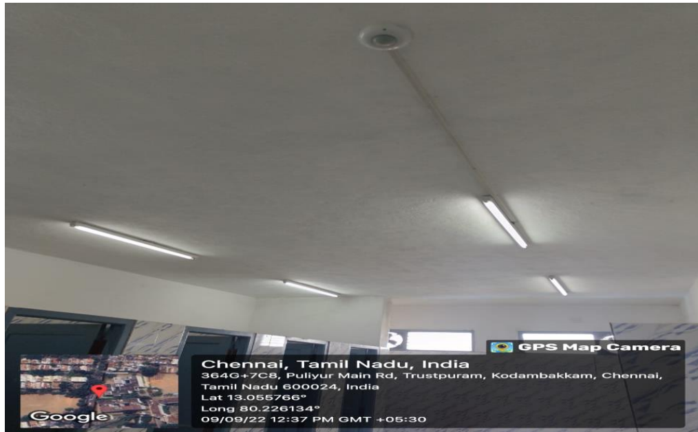
Figure 2. Installed Sensor based Lights in Restroom(Main block)
