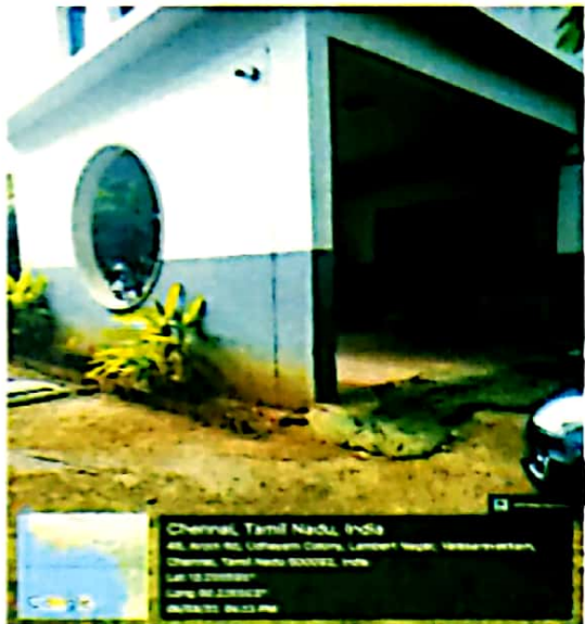
vii) CCTV Camera near parking zone
