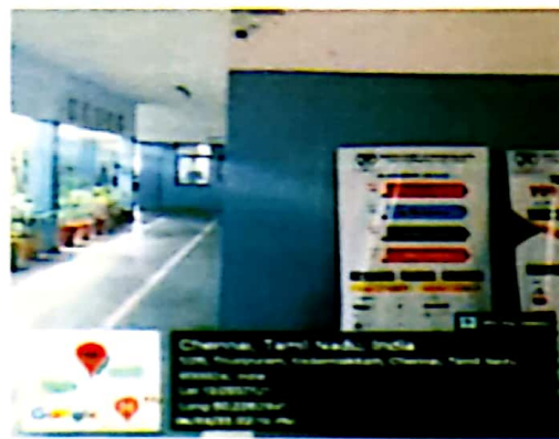
ii) CCTV Camera at Main Building
