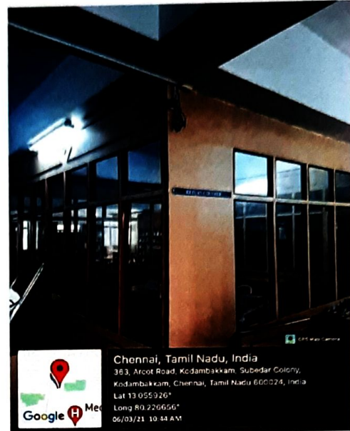
Fig. 6. : CCTV Camera at Library
